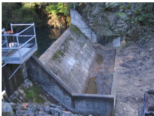
Low Head Dam engineered to control water flow.
