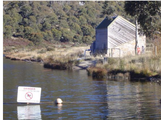
Typical rural pumphouse.
