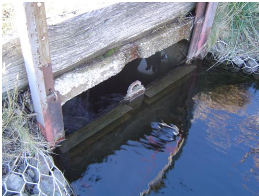
A typical rural spillway.
